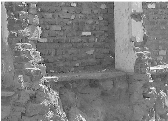
Figure 6: Non-engineered construction: Wall section of a Bachhau residence with burnt clay bricks and mud mortar, widely used before the earthquake. (Source: Photograph by author)
